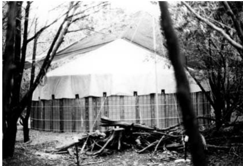
*This 10,700-gallon tank was home-built by Mike McElveen from a stock panel form and sheet metal. Lined with polyethylene film, it stores rainwater for residential use.*
