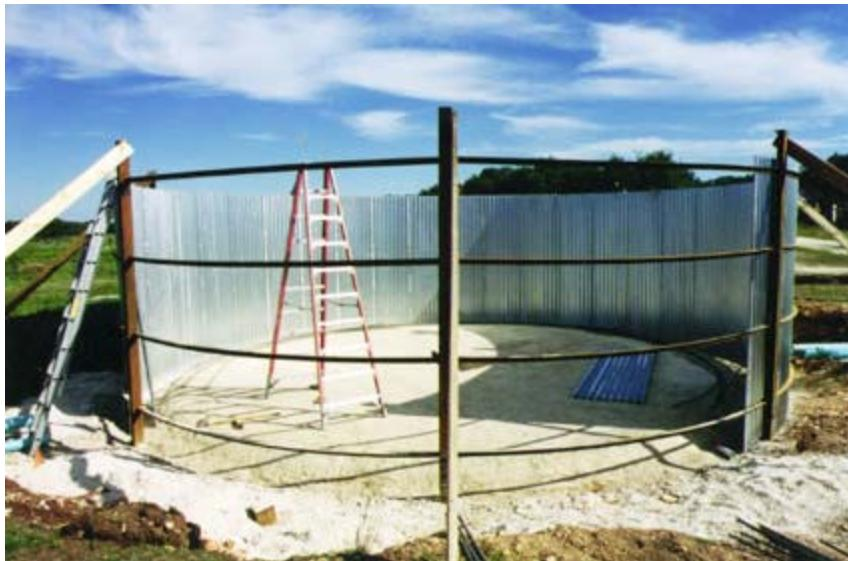
*To construct this 40,000-gallon tank at Avera Armadillo Acres, Sustainable Homesteads first bolted together a frame, then mounted galvanized steel panels to the frame.*
