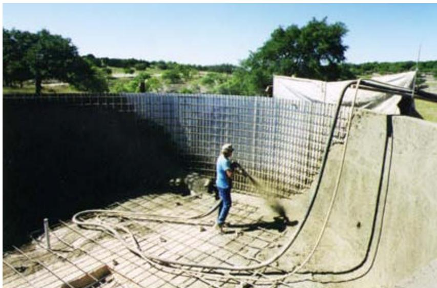
*A proprietary concrete is sprayed monolithically over re-bar to form the inside of the main cistern at Avera Armadillo Acres.*
