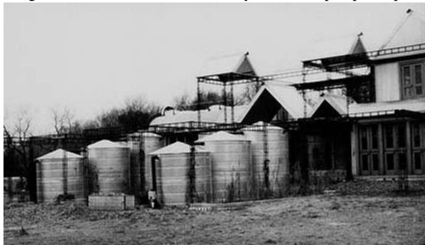
*Galvanized steel tanks, integrated into the aesthetics of this demonstration home, provide 13,700 gallons of rainwater storage at the Center for Maximum Potential Building Systems.*
