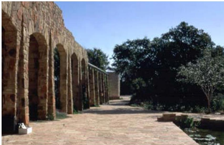
*At the National Wildflower Research Center in Austin, a network of aqueducts conveys water from collection surfaces to cisterns. The 6,000-gallon Entry Cistern shown here is connected to a drip irrigation system.*
