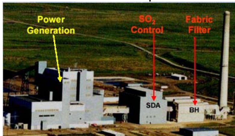
Figure 4: Power plant with semi-dry scrubber for sulfur dioxide control and fabric filter for particulate control
