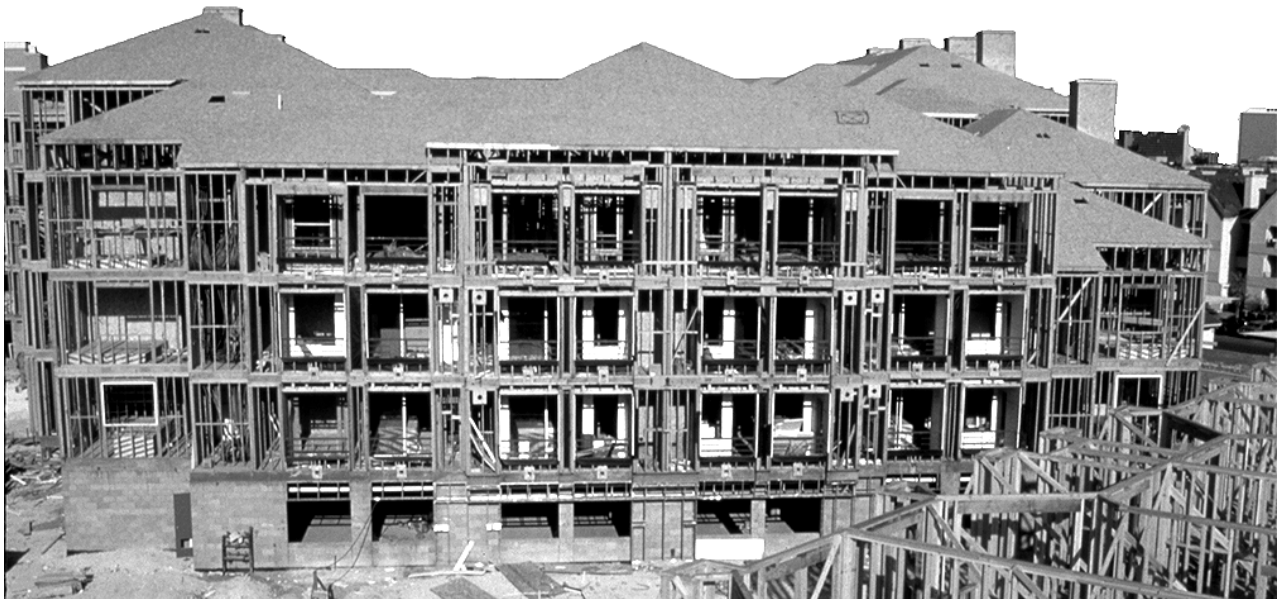
Figure 1. Construction photo of a multi-story wood-frame building
