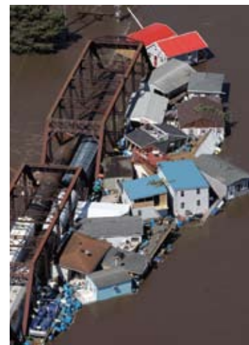
Buildings and debris float up against a railroad bridge on the Cedar River during record flooding in June 2008, in Cedar Rapids, Iowa.
