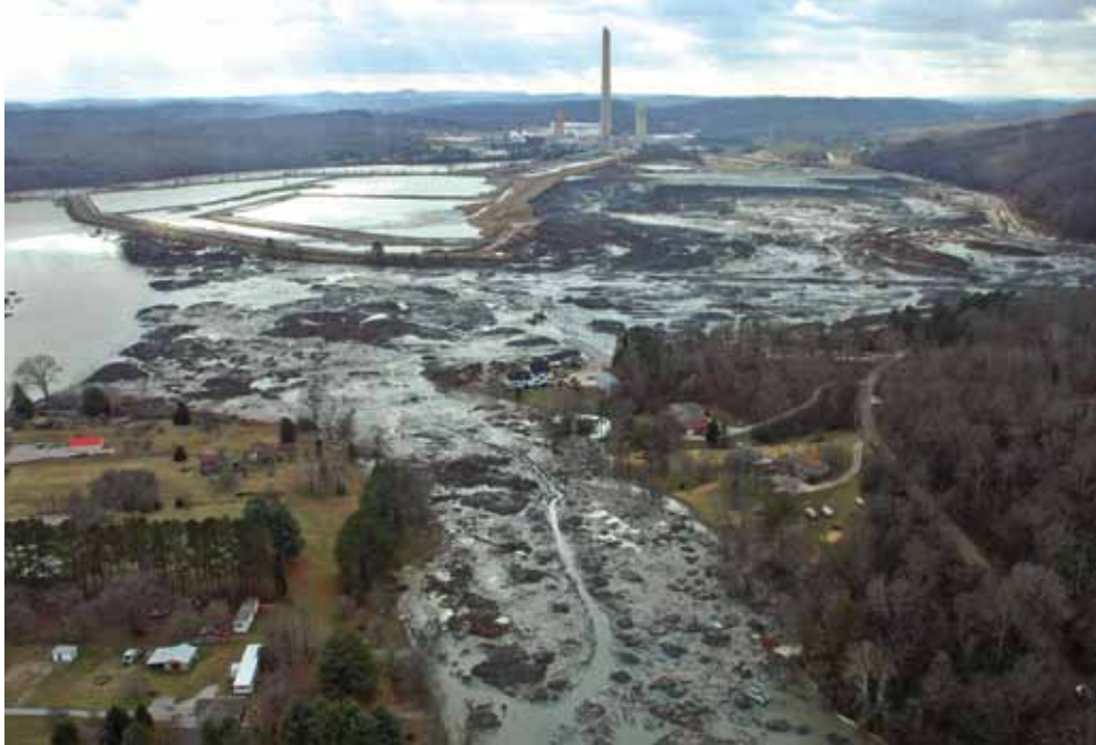
Kingston Fossil Plant—Aerial View of Coal Ash Spill
