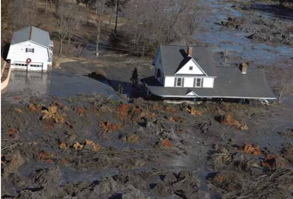
Home destroyed by the Kingston coal ash spill, J. Miles Cary/ Knoxville News Sentinel
