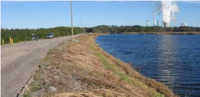
A surface impoundment in Alabama.
