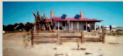
Pueblo of Laguna Solar Electric
