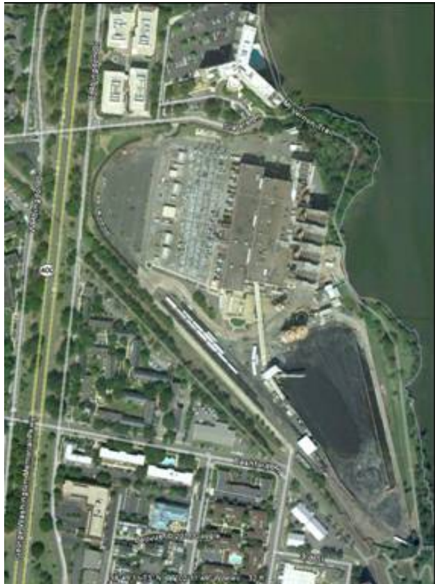
Figure 1 – GenOn Power Plant Site
